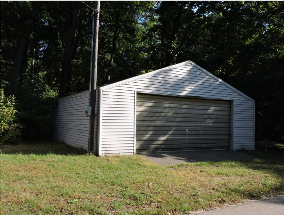
Garage located on back lots across the street from lakefront cottage.
